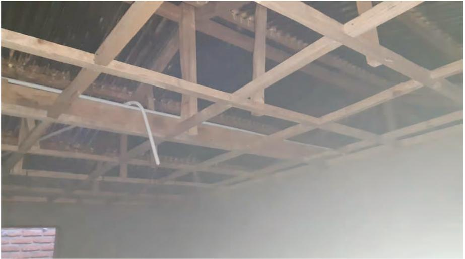
Figure 13: Ceiling structure on hostel houses /Source: Chingalire 2022
